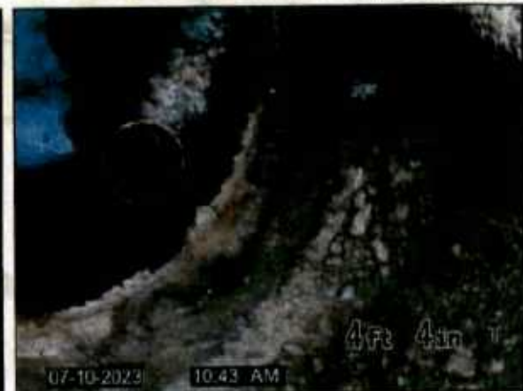
12.1 Item 8(Picture) Line scoped from tank to leachfield
